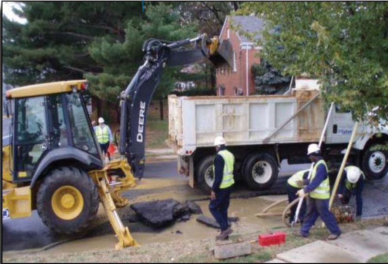
A Fairfax Water crew repairs a main break on Brandon Avenue.
